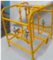
LPG Manifold / Pipelines – Signal red band on canary yellow
