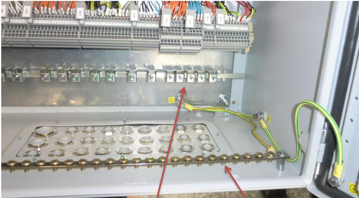
Figure 7 Example of 360-degree earthing.
