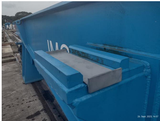
Photo-3: Keel beam lock
