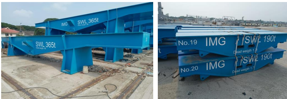
Photo-1: Trestles & keel beams delivered at ISRF site
