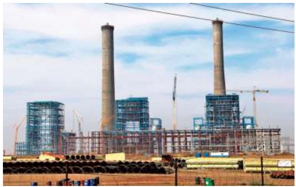
The high operating conditions to maintain an ultra-supercritical plant requires expensive metals and alloys, leading to higher costs
