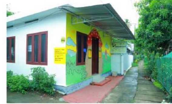
Enhancing Rural Sanitation: Upgraded Facilities for 50 Families in Karumallur, Aluva.
